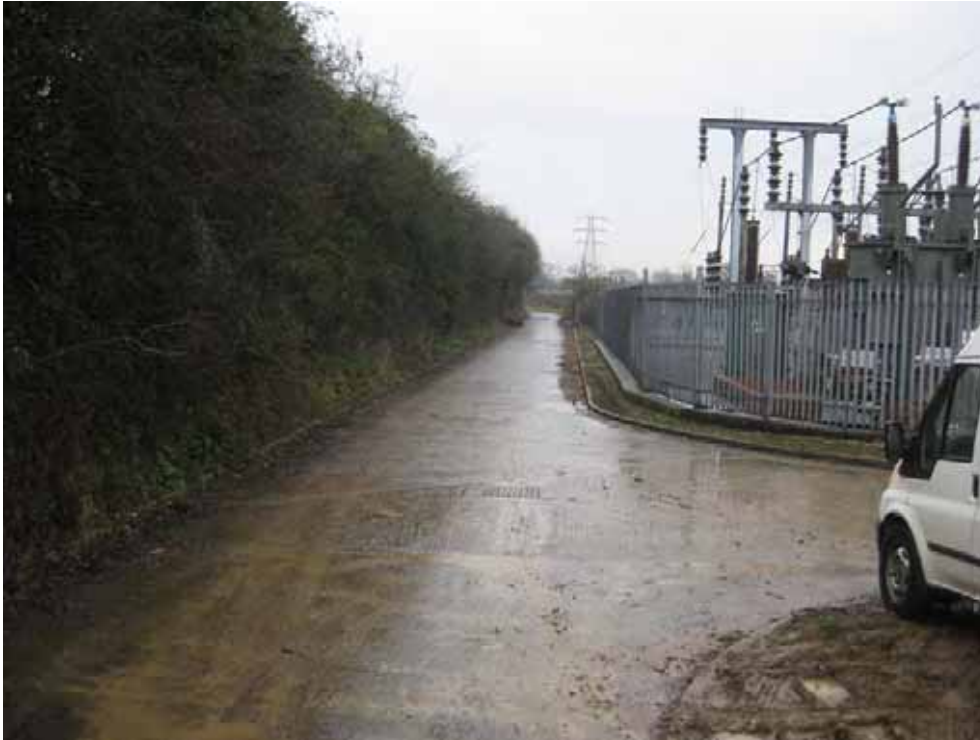
Plate 15 – Facing southeast, a road allowing vehicle access to the east of the sub station.
