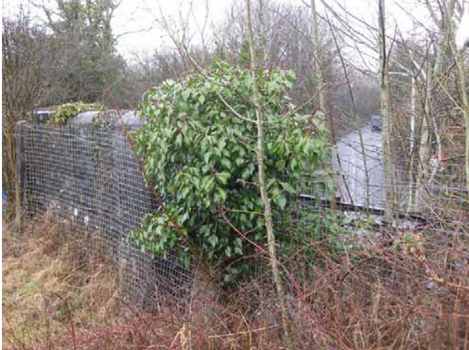
Plate 21 – Facing northeast, the site crosses over Wind Mill Lane.
