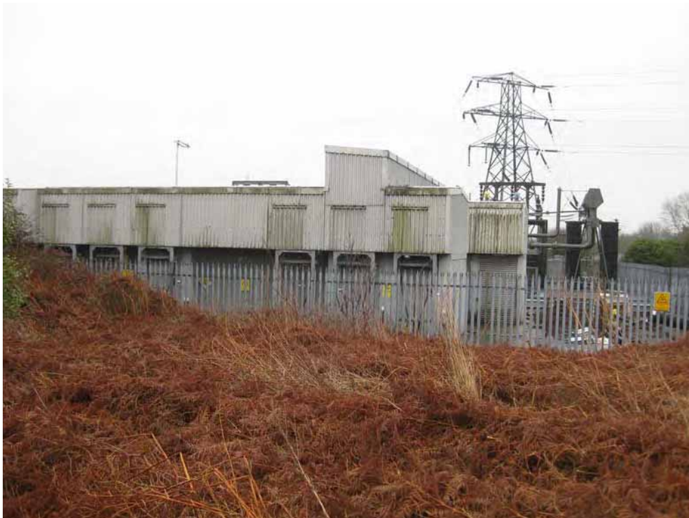
Plate 14 – Facing south, back of the sub-station.
