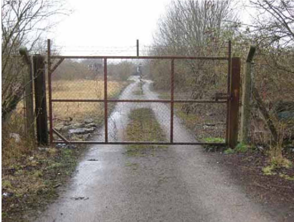
Plate 9 – Facing northwest, another gate and fence crosses the road preventing any further access to vehicles and pedestrians towards the electricity sub-station.
